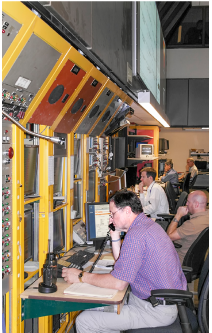
Ray Camp, on the phone, was chief operating engineer; Stephen DePasquale, center, was chief operating engineer in training; and Devon Battaglia, right, was the physics operator, for CD-4. Behind them are engineers John Dong and Nevelle Greenough. (Photos by Jeanne Jackson DeVoe)
