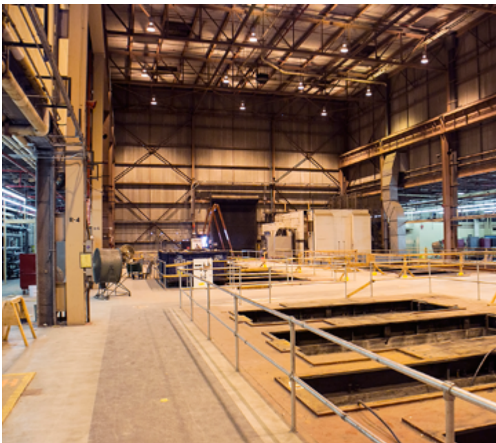
The C Site motor generator building will be renovated to house technical shops.
