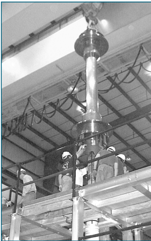
Figure 3. Completed NSTX center stack.
