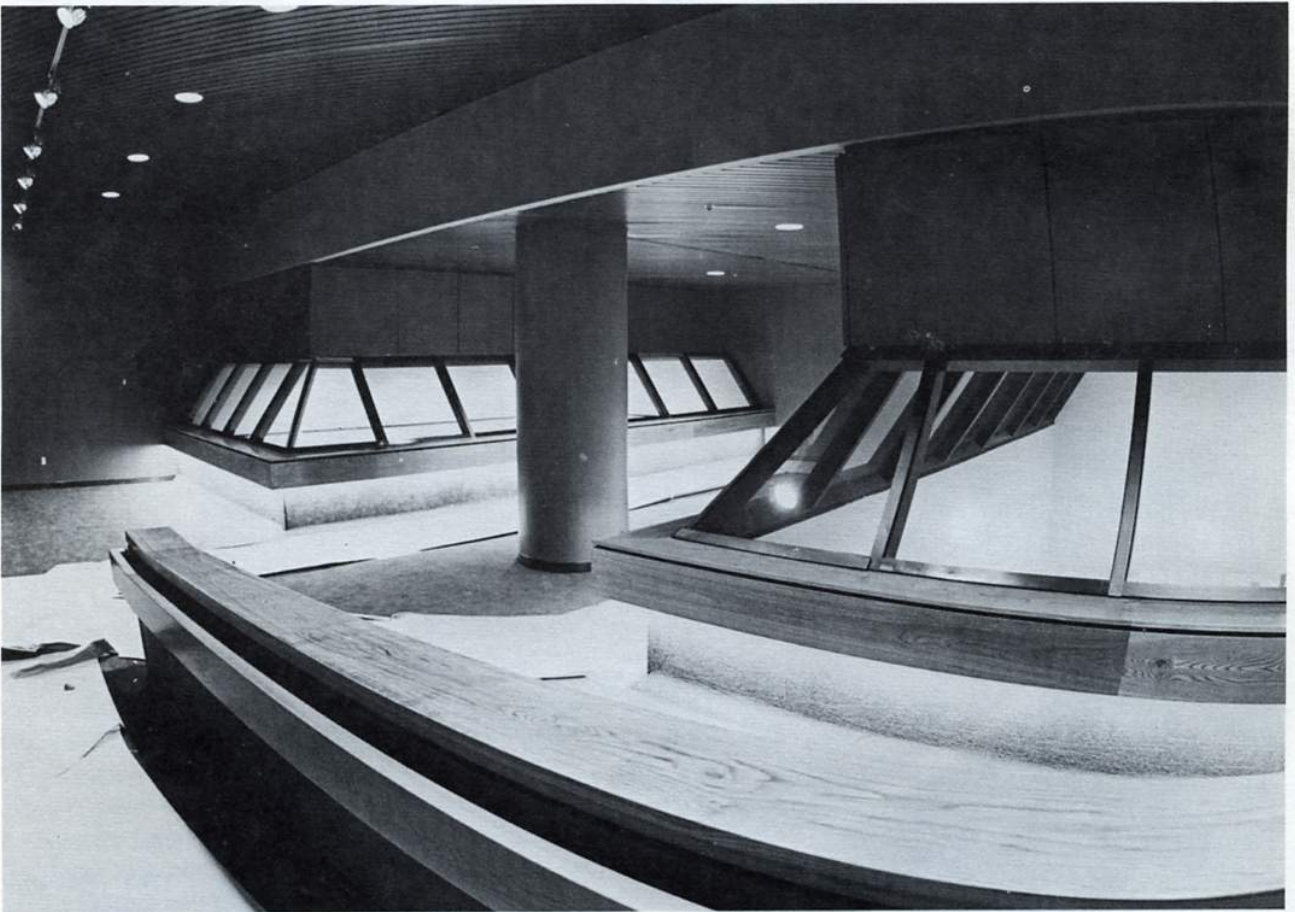
Within the west wing of the Lab/Office Building, the TFTR visitors' gallery is complete. The windowed viewing area on the left overlooks the TFTR control room; the one on the right overlooks the computer room.
