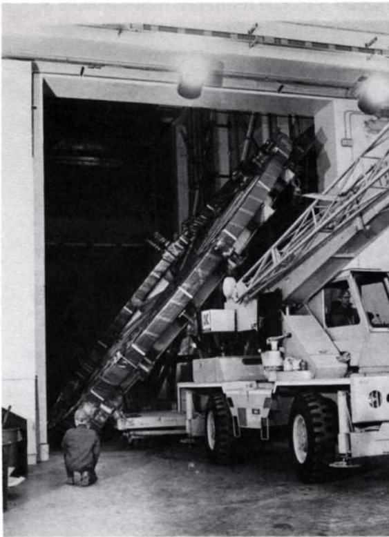
Despite the rather tight fit, the coil was safely moved through a second doorway connecting the mockup area with the test cell.
