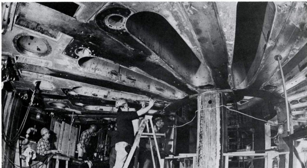
Large racetrack-like openings provide diagnostic access from the underside of the six-foot-thick machine base into the TFTR vacuum vessel. The wide angle shot shown above distorts the machine geometry.
