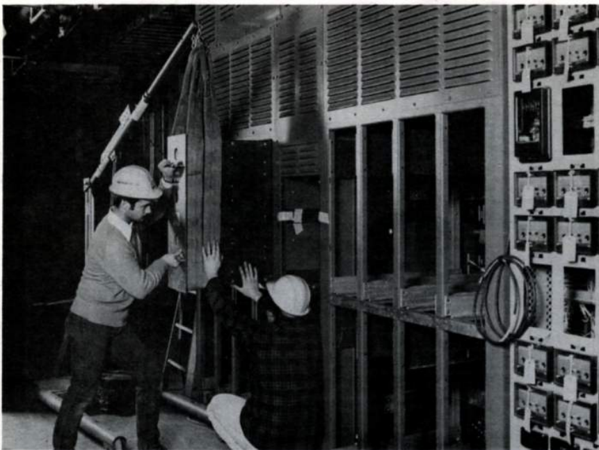
Pete Haney (standing) and John Opperman guide another TFTR rectifier component into place. Seven rectifiers were recently run in series, with power provided by the TFTR MG set.
