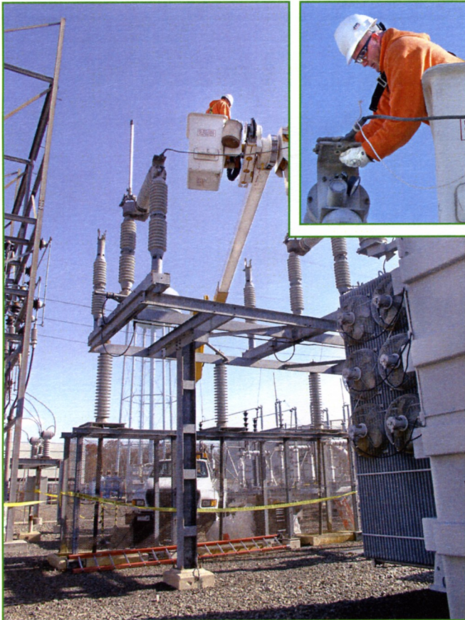
Bill Burchill disconnects an old switch in the switch yard.
