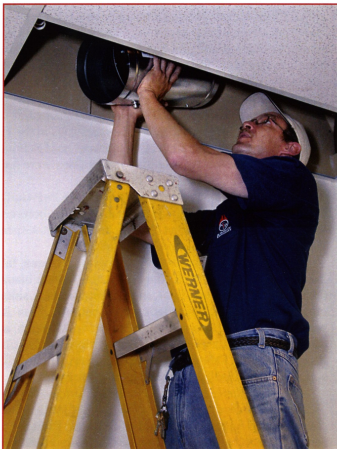
Kevin Taylor of Master Fire Protection installs a damper for the Variable Air Volume Air Handling Unit upgrade in a Lyman Spitzer Building office. When the project is completed, 87 zones will have new units, leading to greater energy efficiency.
