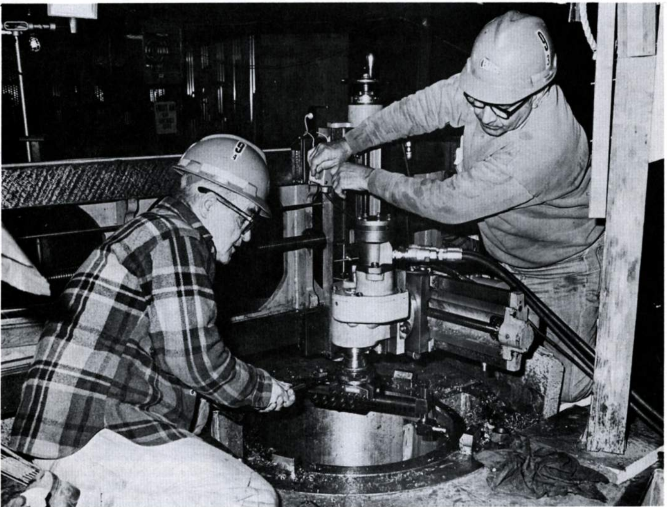
Workmen are machining the central plug that will serve as a base for the TFTR central column.
