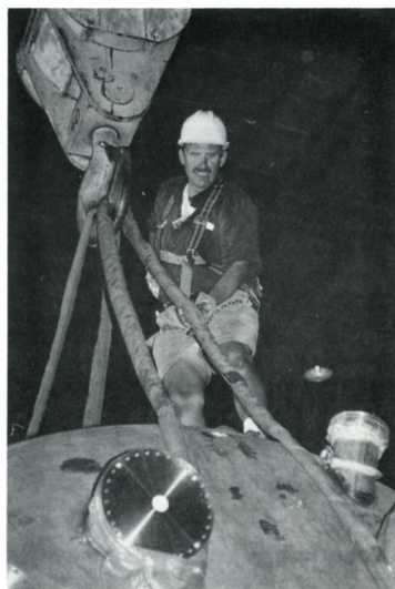
PPPL's Joe Bartzak assists with the rigging of the National Spherical Torus Experiment (NSTX) vacuum vessel in preparation for lifting the vessel off the delivery truck and into the RESA building. NSTX is now under construction at PPPL and is being built jointly by PPPL, the Oak Ridge National Laboratory, Columbia University, and the University of Washington at Seattle. PPPL has primary responsibility for the Project. See photo essay about the arrival of the vacuum vessel on pages 5 and 6.
