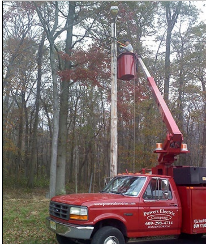
Workers repair lights outside the LSB lobby, where an electric line to streetlights was damaged.
