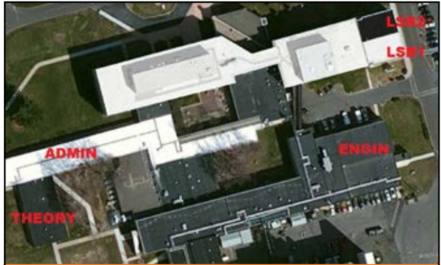
A revised overhead photo of the black and white roofs installed on PPPL buildings as part of the cool roofs project. (Photo courtesy of Mark Hughes).
