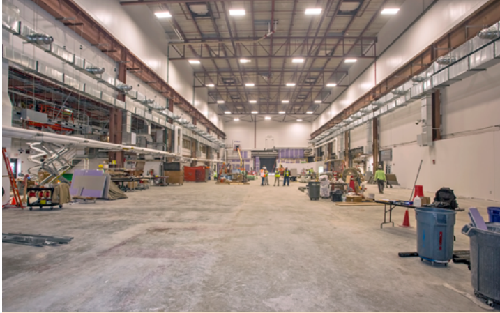
View indicating the length of the C Site-MG Building. (Photo by Elle Starkman)
