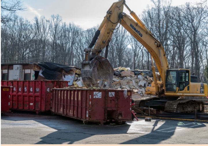
The excavator removes building materials. (Photo by Elle Starkman)
