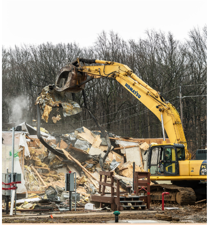
An excavator tears into the Mod 6 building. (Photo by Elle Starkman)
