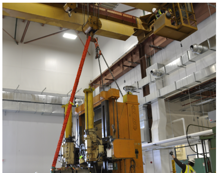
A crane lifts the King Machine. (Photo by Ken Bauer)
