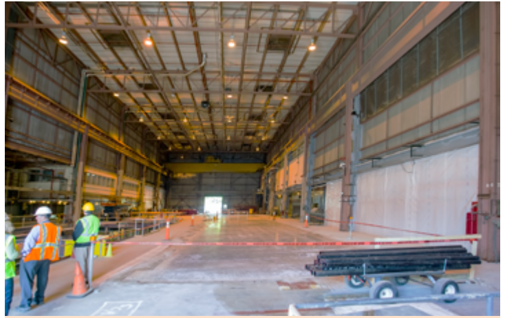
The new concrete deck in the C-Site MG Building. (Photo by Elle Starkman)
