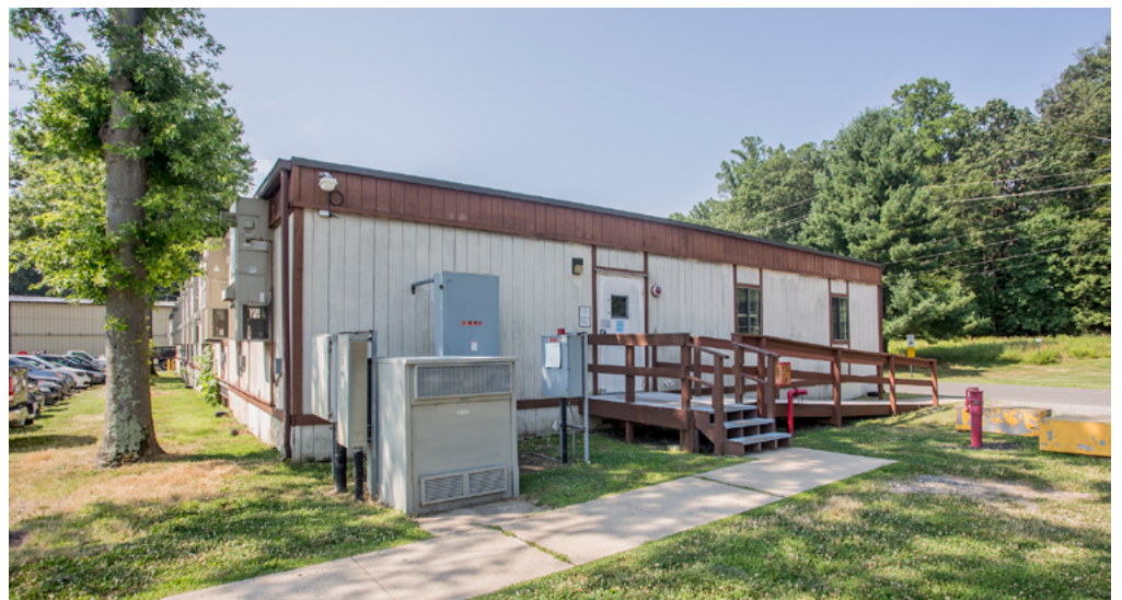
The second phase of the IOI construction plan calls for the demolition of Mod 6. (Photo by Elle Starkman)
