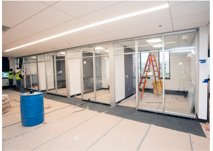
Glass partitioned offices on the first floor of the LSB Annex. (Photo by Elle Starkman)
