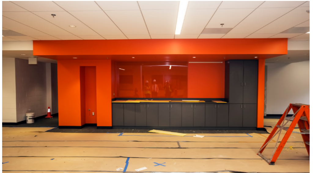
The back wall of the LSB Annex third floor. (Photo by Elle Starkman)
