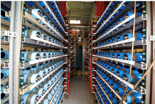
Figure 3. Photo of the full ohmic power supply. The original capacitor bank is to the left, the new bank is to the right. The IGBT-based H-bridges and the buswork are at the far end of the capacitor banks.
