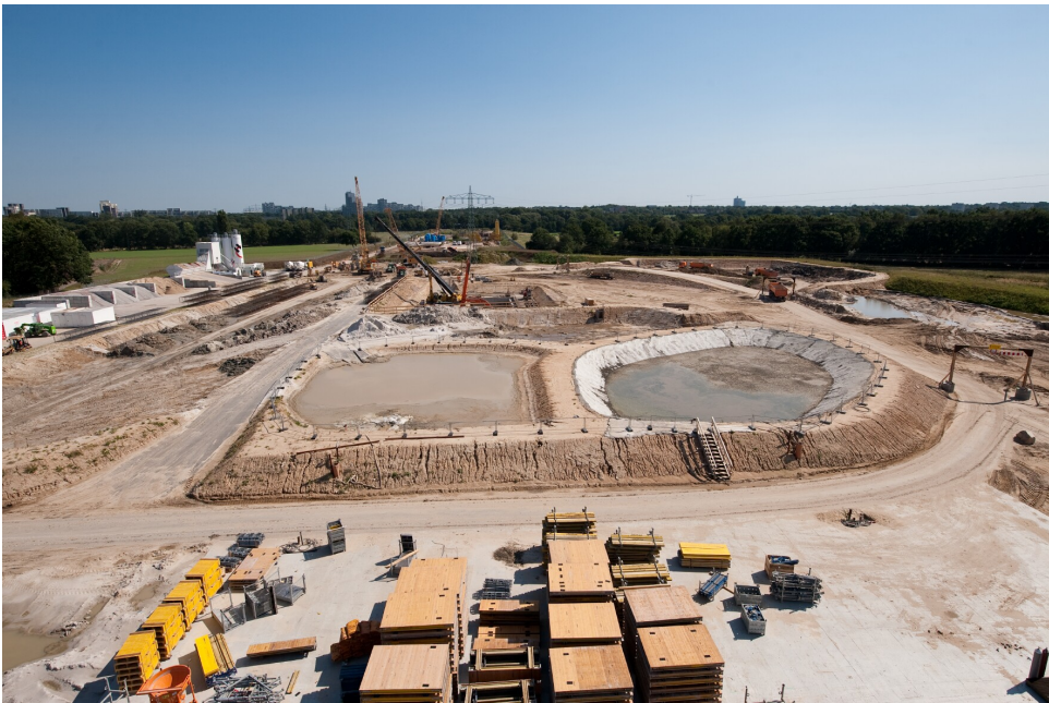
XFEL construction site: 9/1/09
