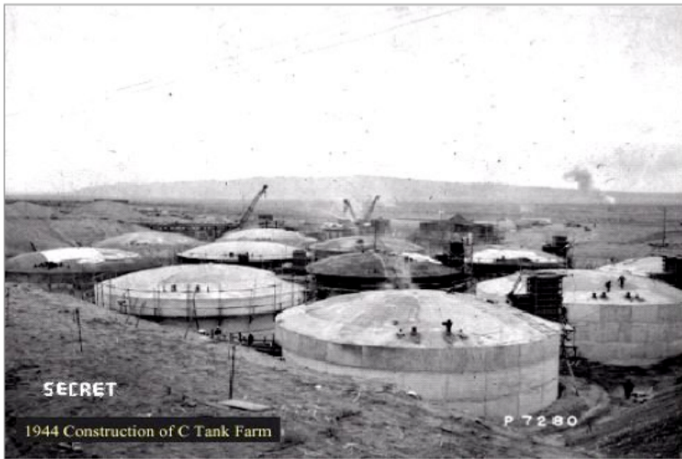
Single shell tanks constructed in 1944
