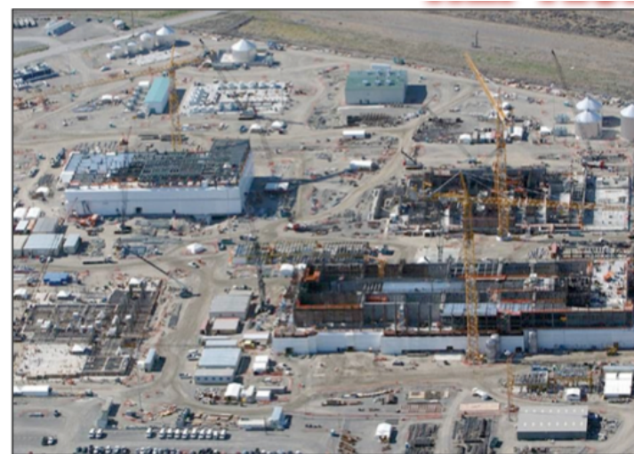
Waste treatment plant in 2005
