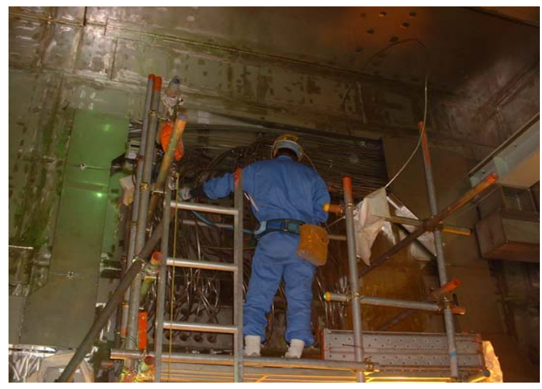
Laying operation of MI cable which penetrates the wall
