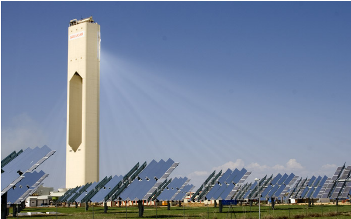
Figure 5 – “PS10”, 11MW (2004), located in Seville, Spain
