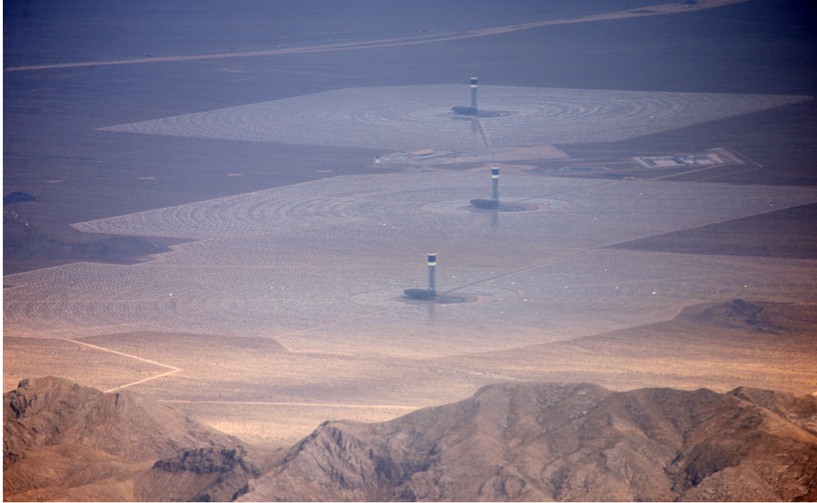
Figure 4 – “Ivanpah”, worlds largest CSP facility, 392MW (2014), located in Mojave Desert, California, USA
