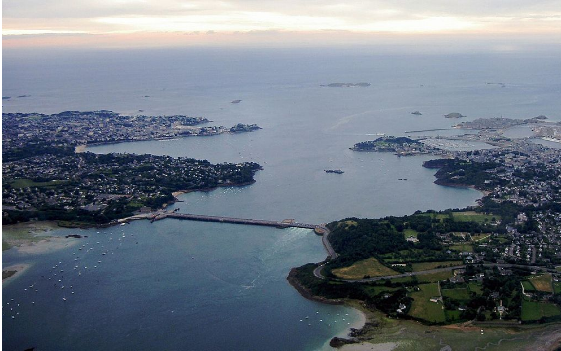
Figure 12 – Rance Tidal Power Station, 24 generators @ 10MW, total 240MW (1967), located in Brittany, France
