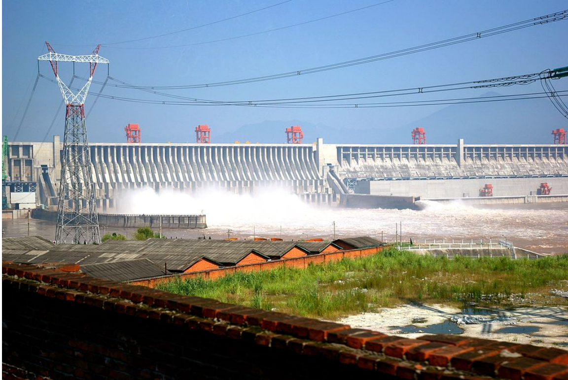
Figure 24 – “Three Gorges”, World’s Largest Reservoir Hydroelectric Power Plant, 32 generators @ 700MW, total 22.5 GW (2012), Yangtze River, China
