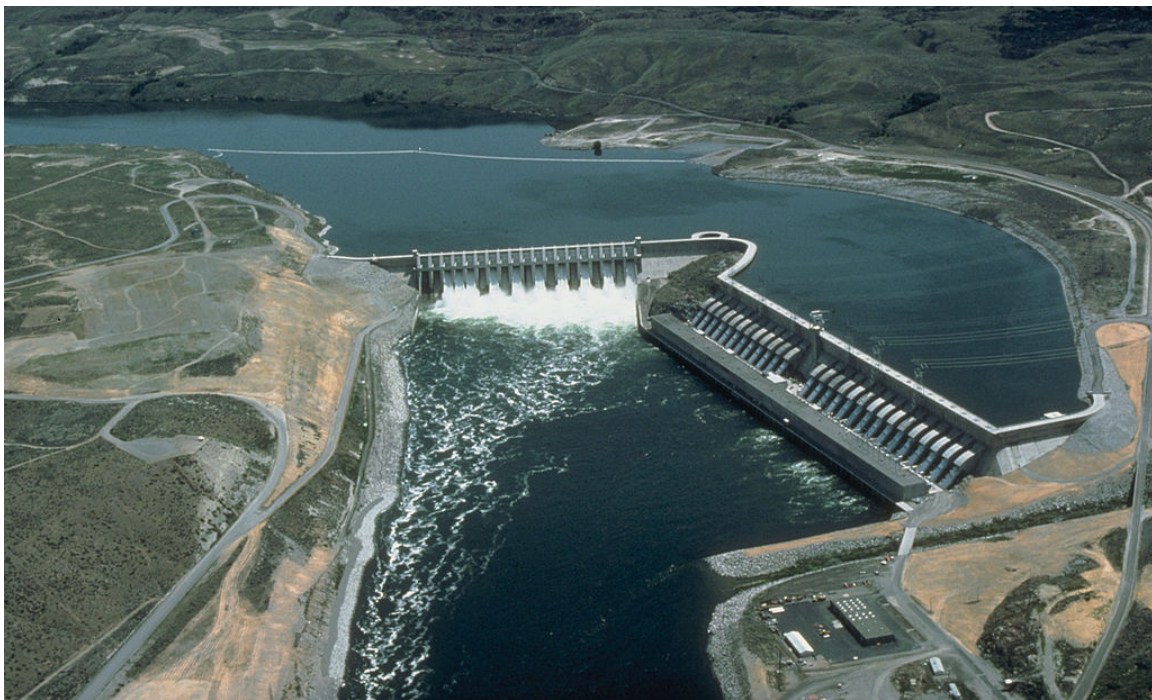
Figure 25 - “Chief Joseph Dam”, World’s Largest Run-of-River Hydroelectric Power Plant,
