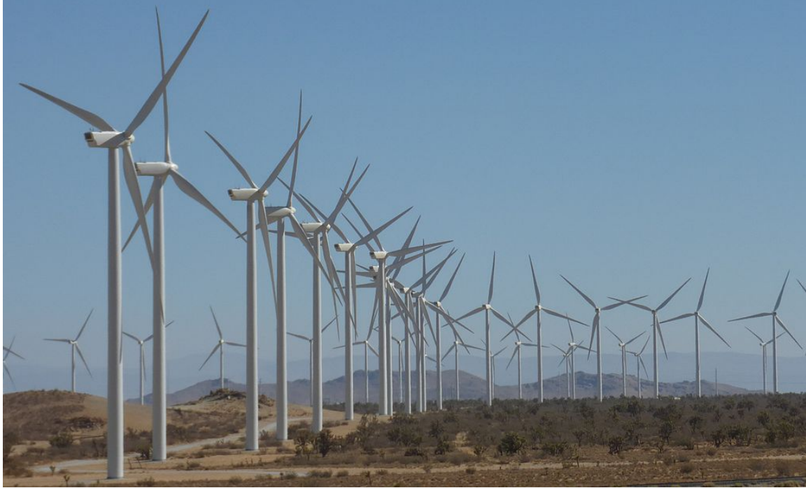
Figure 15 – World’s Largest Wind Farm – “Alta Wind Energy Center”, 490 turbines, 1320 MW (2011), Tehachapi Pass, California, USA
