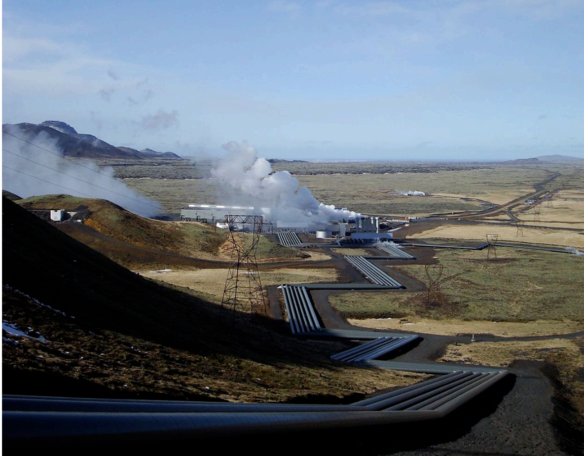
Figure 20 – “Hellisheiði” Power Station, 50 wells, 7 generators, 300MW (2006), located in Hengill, Iceland
