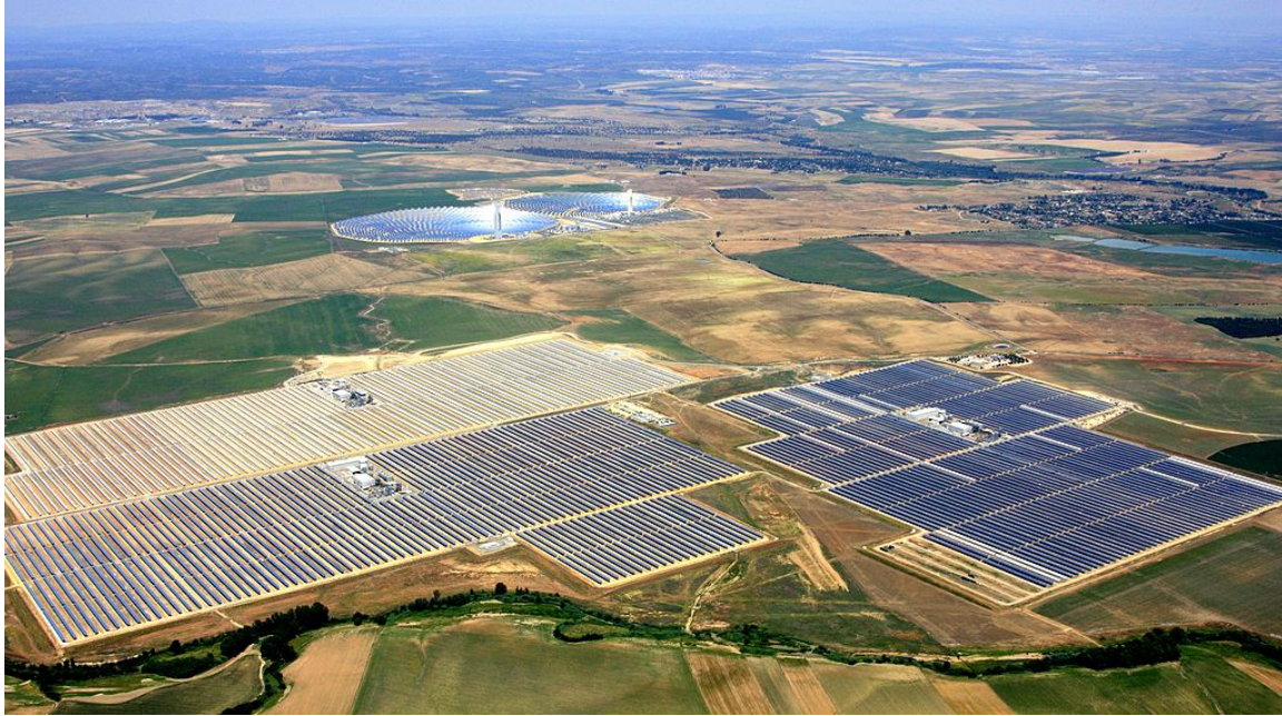
Figure 6 – “Solnova”, 250MW (2014), Seville, Spain
