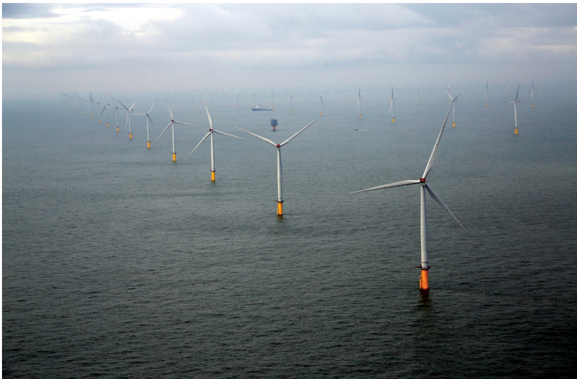
Figure 16 – World’s Largest Offshore Wind Farm – “London Array”, 175 turbines, 630 MW (2011), Thames Estuary, UK
