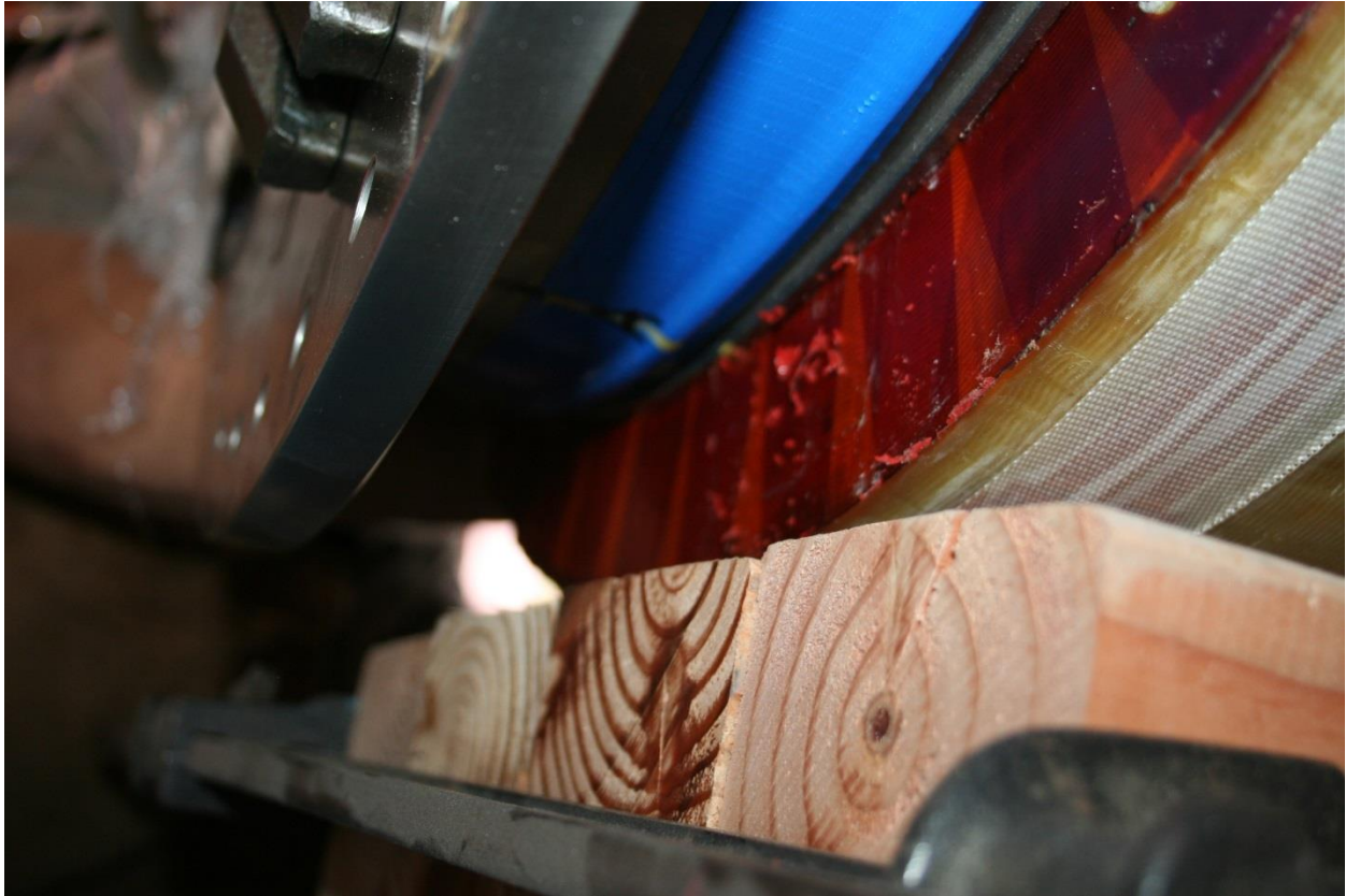
Figure 78 – Coil pack section B_C removal
