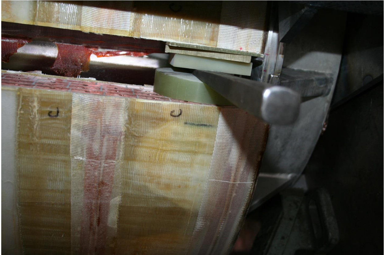
Figure 77 – Coil pack section B_C removal
