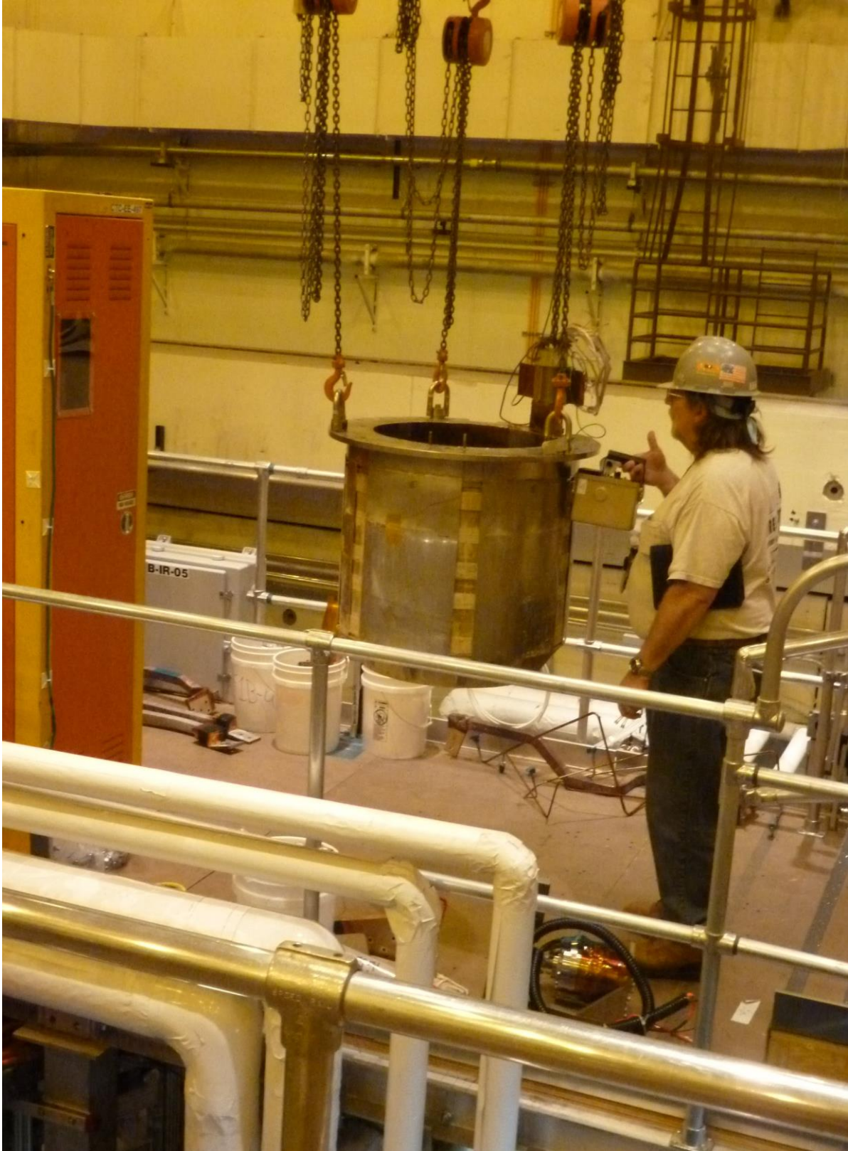
Figure 9 – HP surveying PF1A-U post-removal
