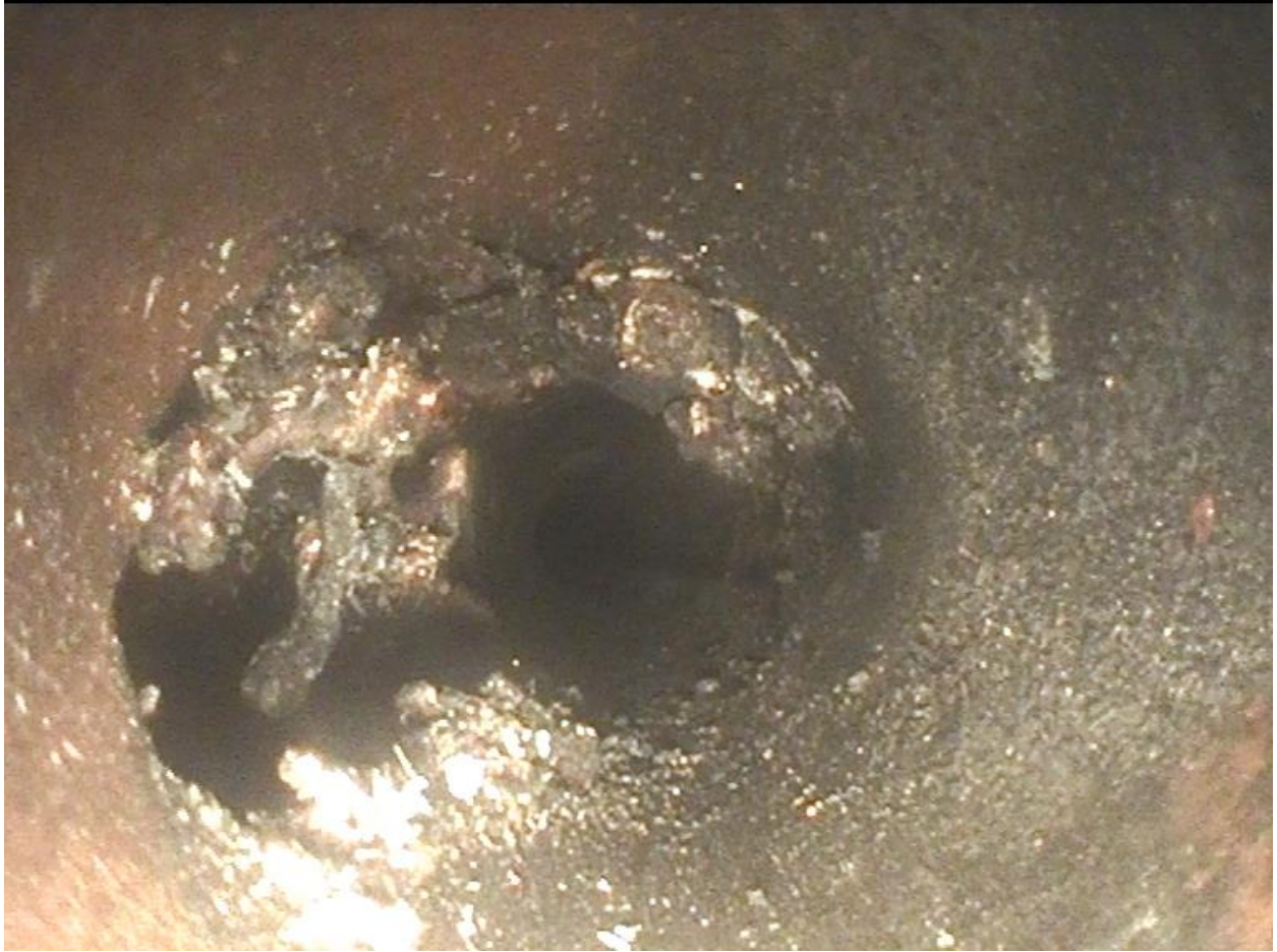
Figure 109 – Void – view from plane A
