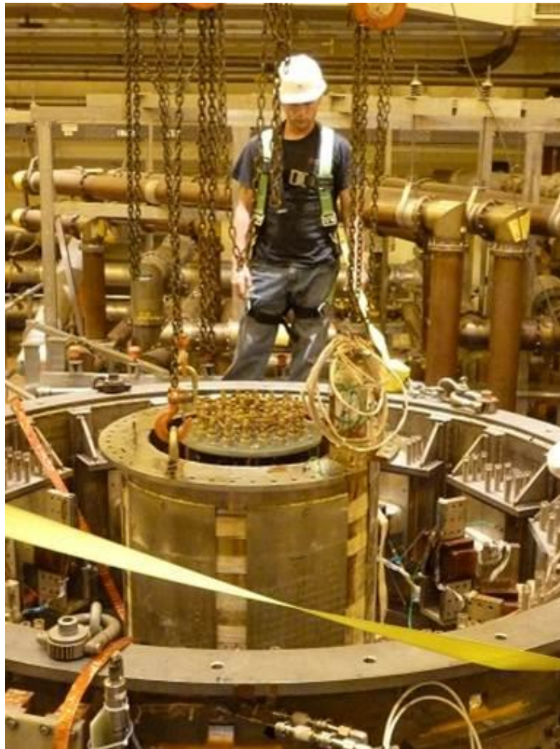
Figure 7 – Removal of PF1A-U from NSTX-U
