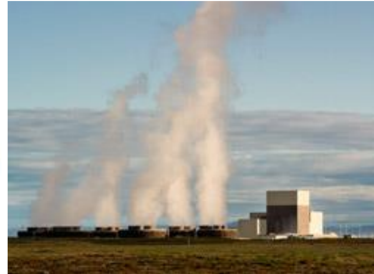
Columbia Generating Station (Richland, WA)
